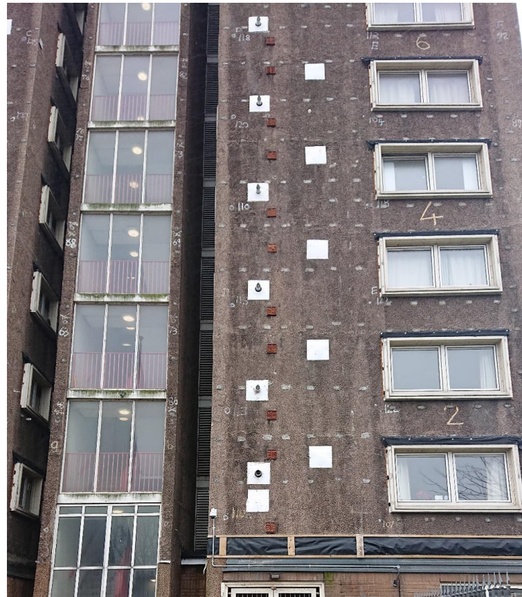
Front of tower block with cladding removed
